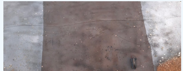
BEFORE Sandblasted white metal. Center coated in S2S
